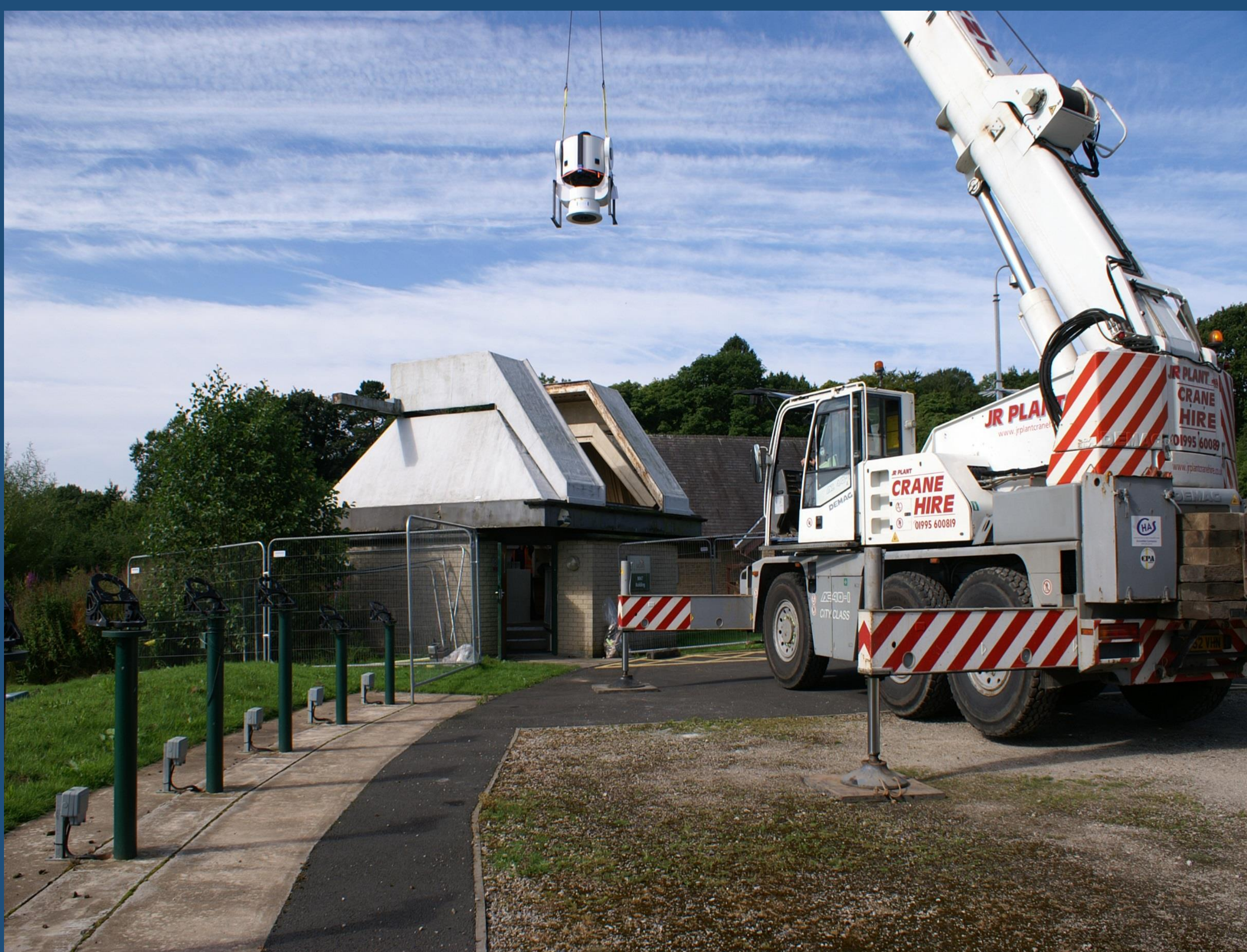
Figure 2: The telescope arrives at Alston. The primary mirror housing and yoke mount are lowered into the building in a single section.
